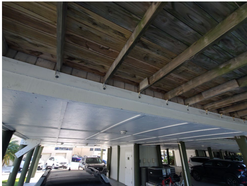
FLOOR JOIST CONNECTION AT PORCH
