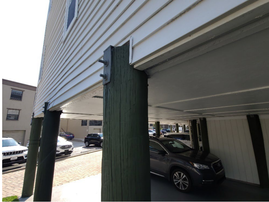
SERIES OF PILES + TOP CONNECTIONS
