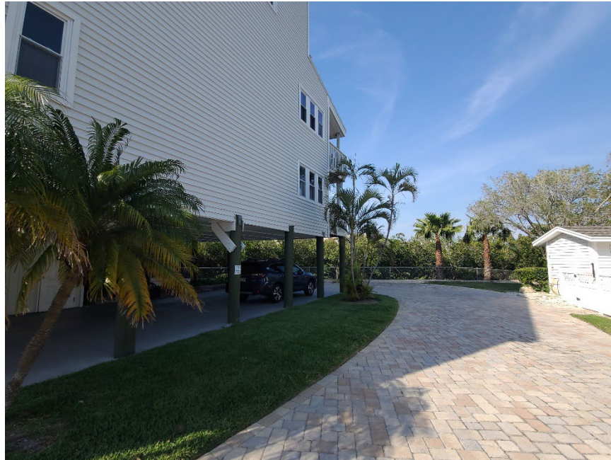
EAST SIDE OF BUILDING + PILE SUPPORT
