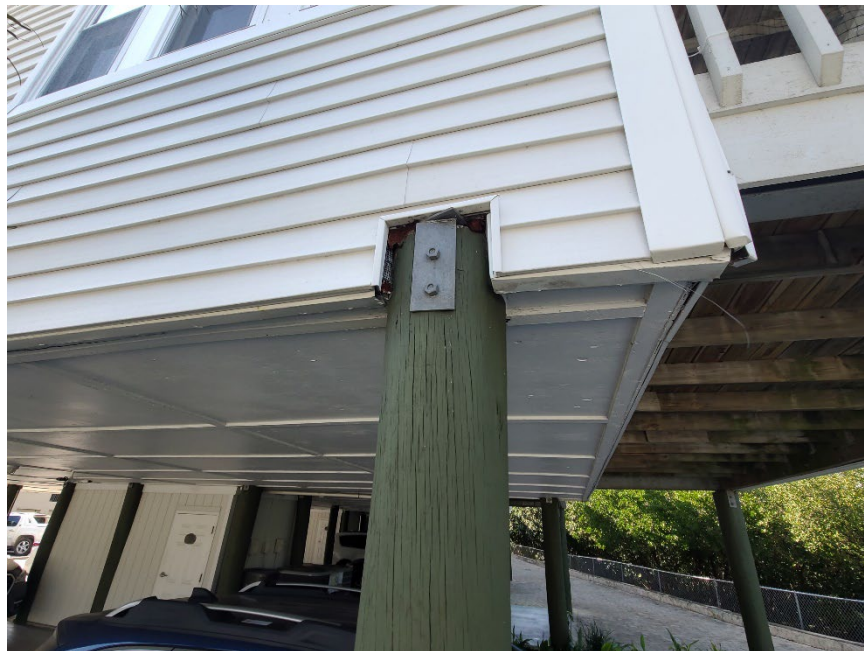
TYPICAL PILE TOP CONNECTION
