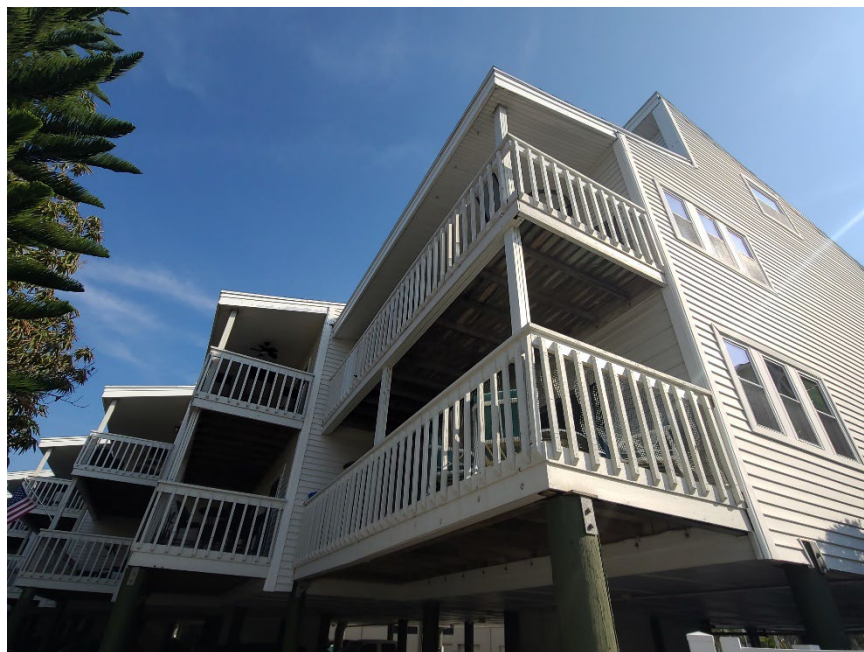
2 ND + 3 RD FLOOR PORCH FRAMING
