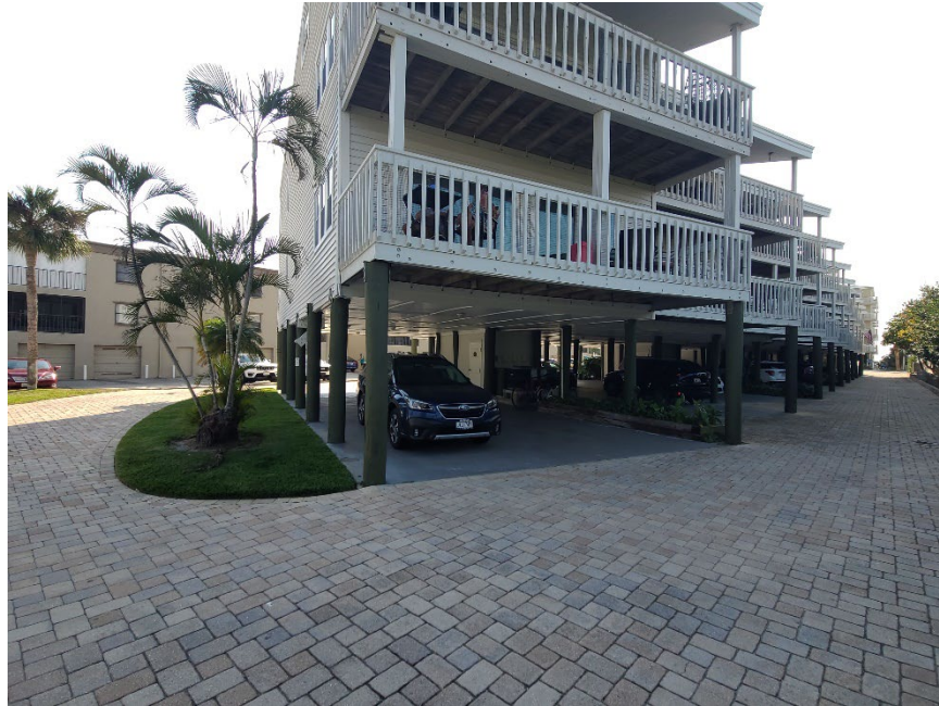
NORTH SIDE OF PROPERTY + PILE SUPPORT
